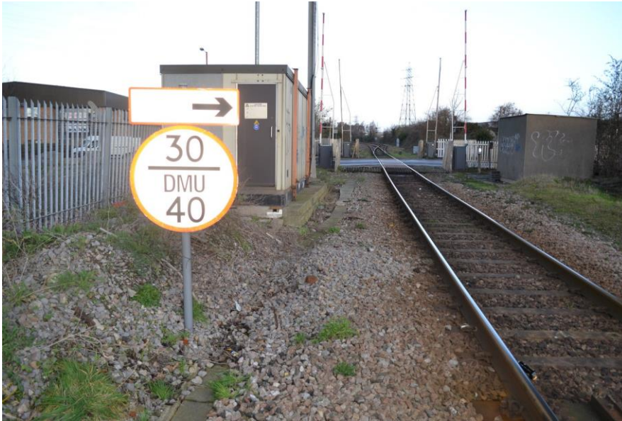
Figure 18 - looking towards high mileage at Avonmouth Dock Level Crossing
