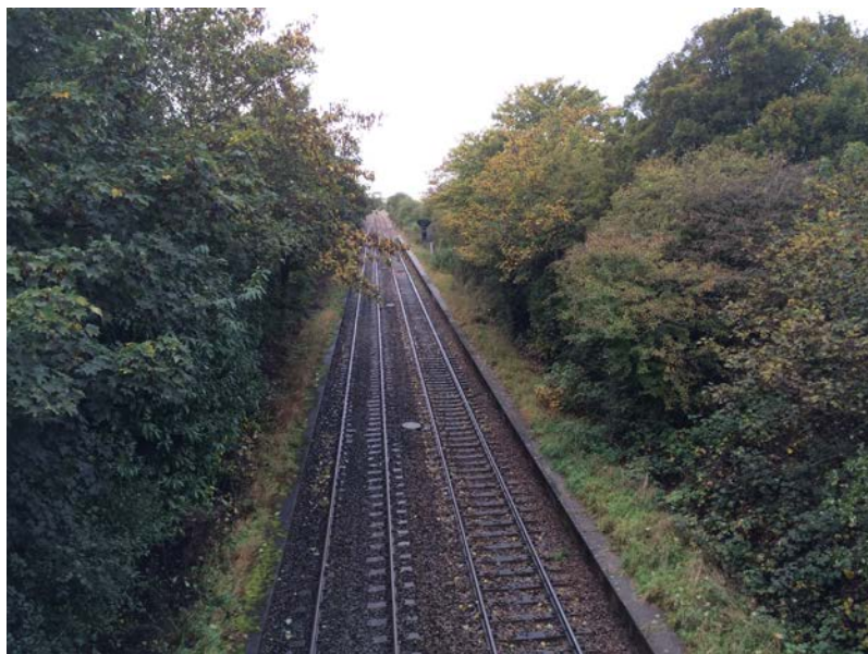
The existing Freight Route – Filton West Junction to Hallen Marsh Junction and the redundant platforms at North Filton
