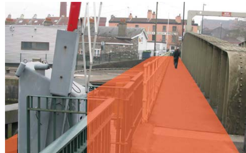
Widened walkway along east side of Cumberland Basin Bridge
