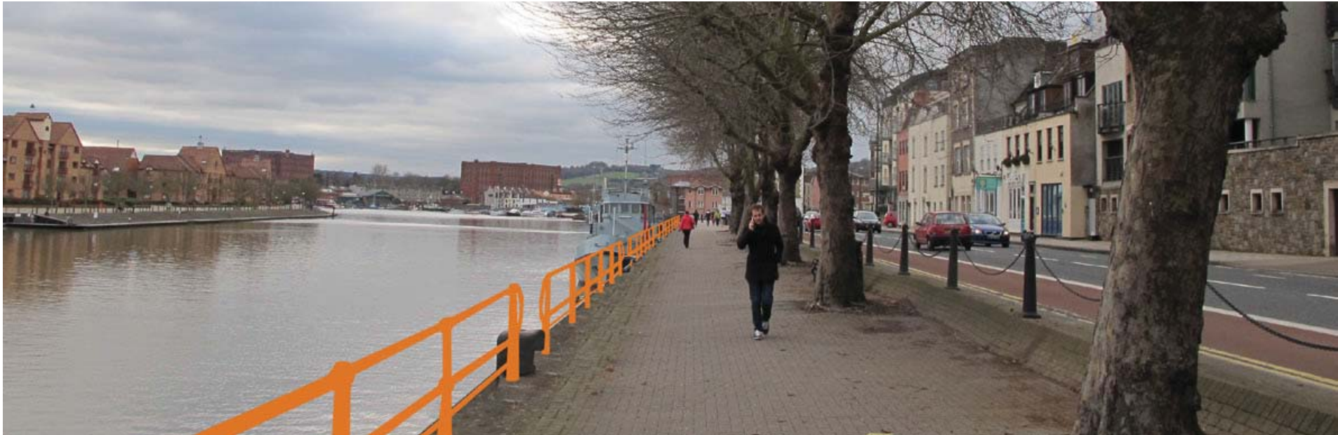
View showing railings moved to gain more space on promenade
