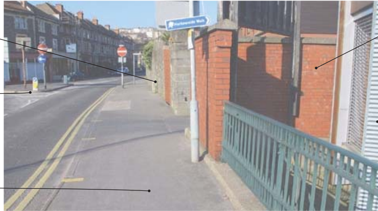
View of approach to Pump House entrance from the Cumberland Basin Bridge
