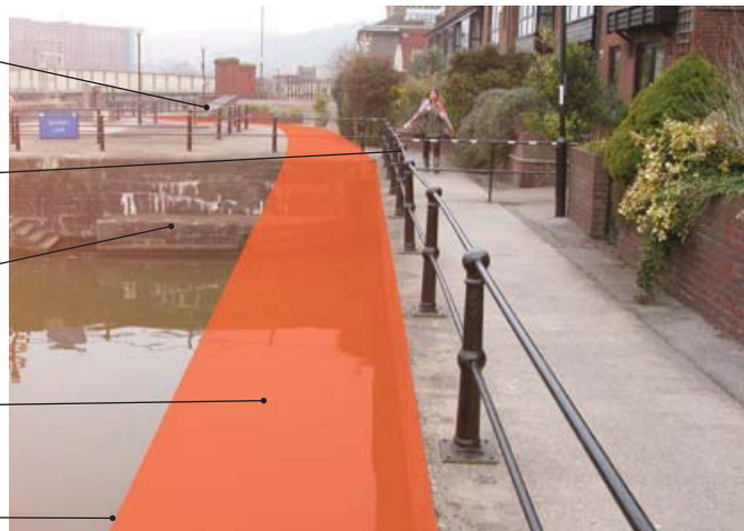
View of Cattle Market Dock entrance where the constructed walkway needs to be augmented
