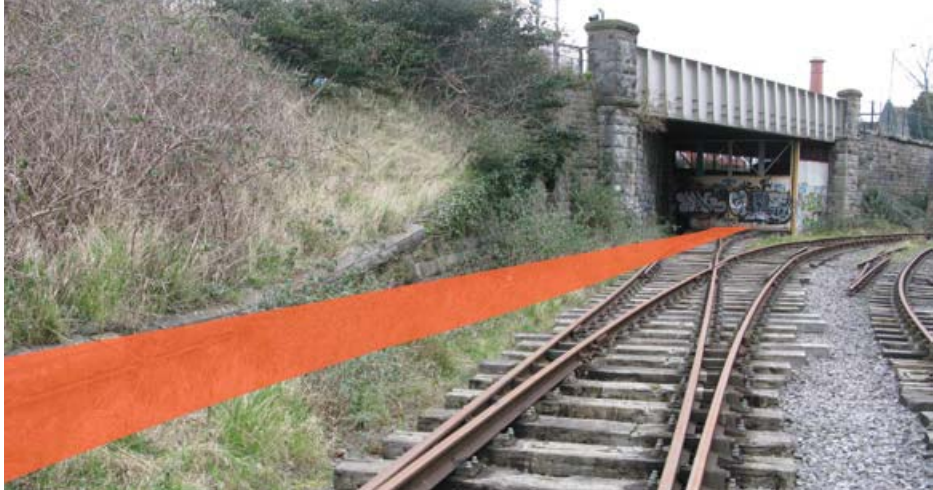
View approaching Cumberland Road Bridge showing route alongside railway
