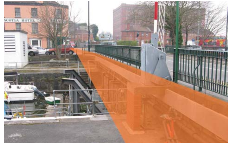
Footpath extension required at Old Junction Lock
