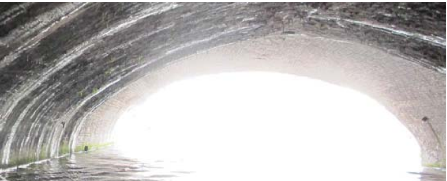
Views of river beneath railway
