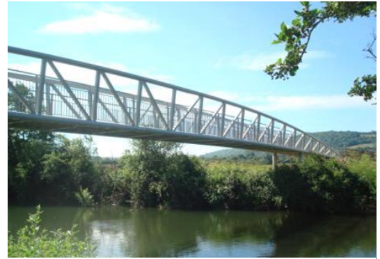
New pedestrian and cycling bridge at Batheaston
