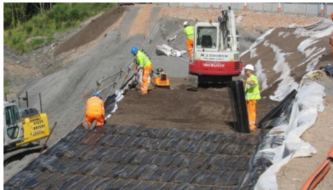
M5 Junction 21 improvements
