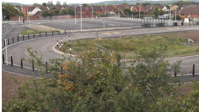
New car parking and interchange at Worle station
