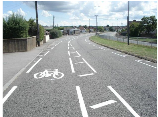
A432 Chipping Sodbury road safety scheme - reduced speed limit, new cycle lane and improved road surface
