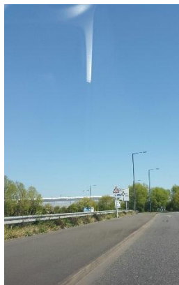
View looking north to Poplar Way junction
